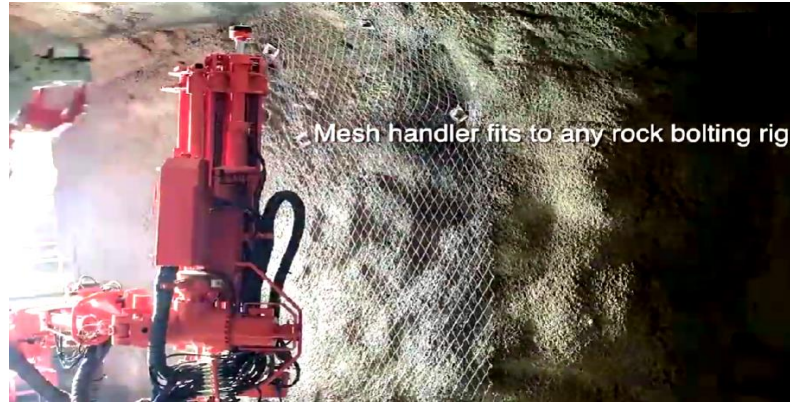
Fig. 2. Mesh handler instalment on the tunnel walls.
