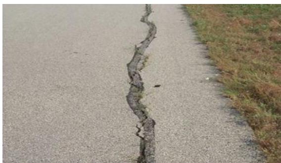
Fig. 3. Roadside fracture.
