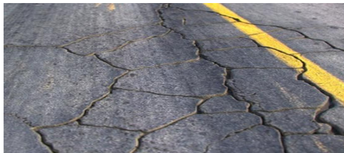
Fig. 5. Shrinkage cracks.
