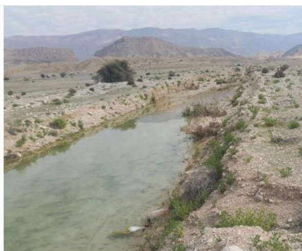
Fig. 3. View of the inlet structure of the Bushkan Plain project.
