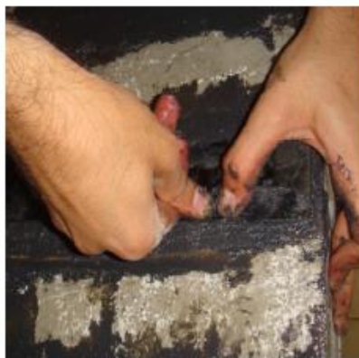
Fig. 2. Installation of FRP fibers over the Resin.
